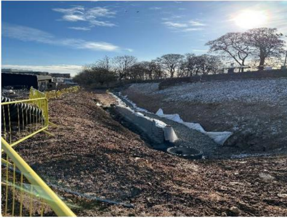
Grid Line 1 retaining wall
