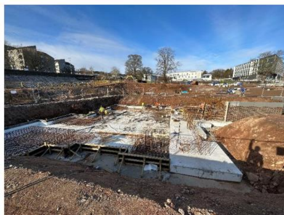
PM room excavations completed with the lower slab 50% completed,
