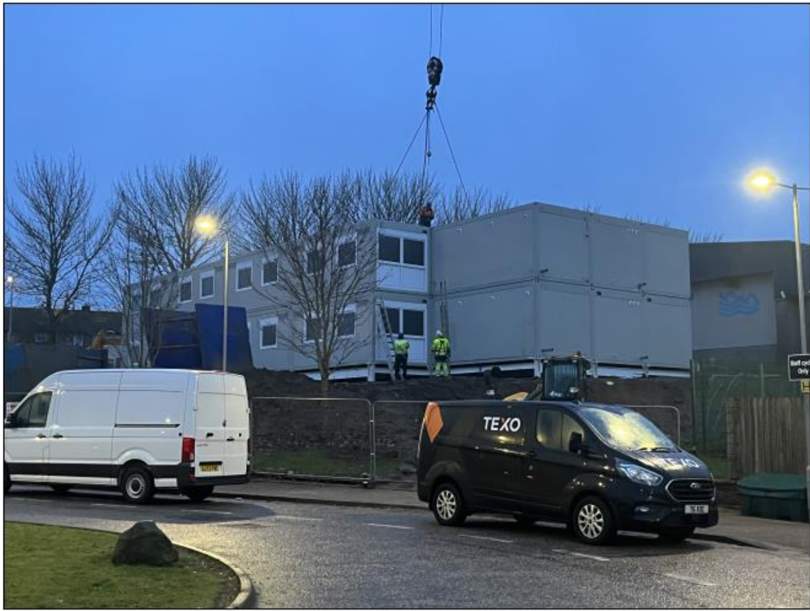
Installation of the units
